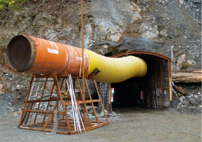
3300 feet (1005.84 meters) Underground Development
