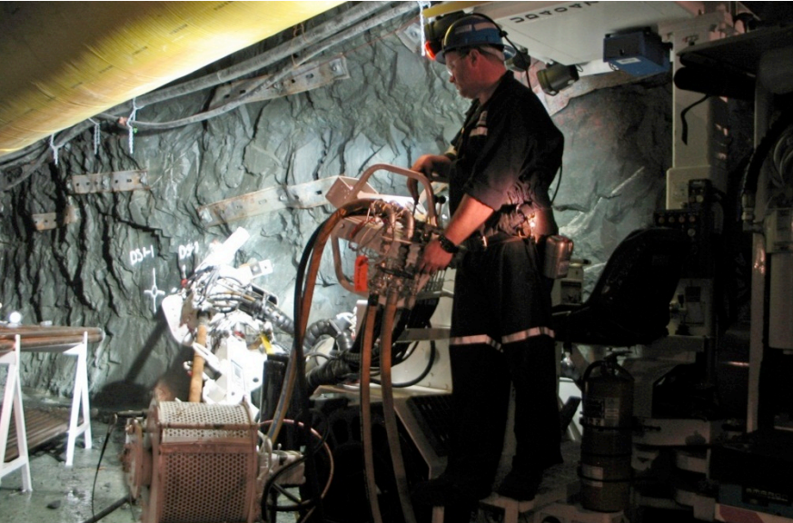
Underground Drilling Year Round
